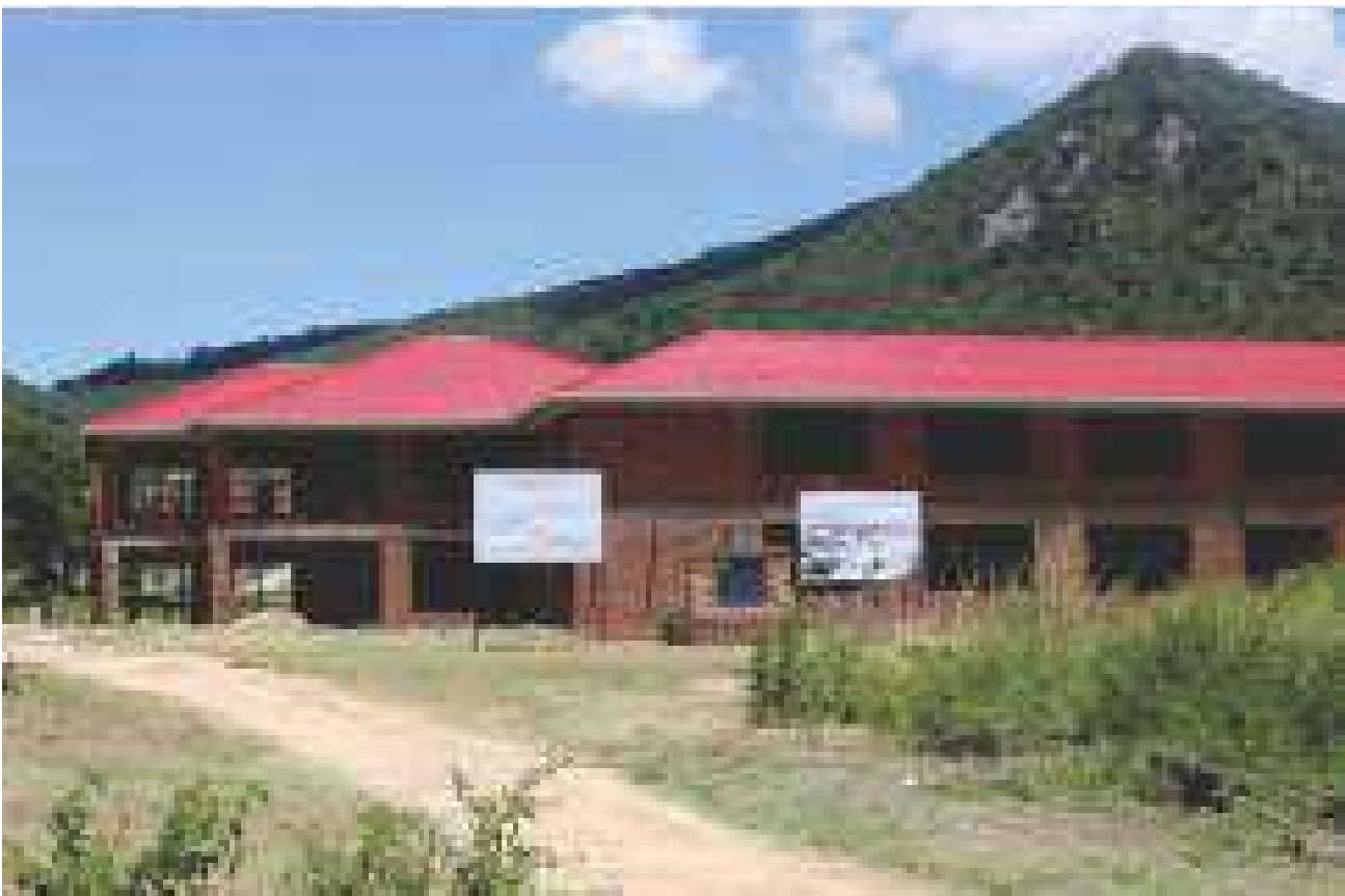
Manicaland State University of Applied Sciences Female Hostel Under Construction
