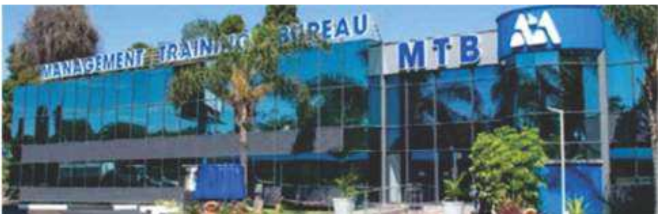
Refurbished Management Training Bureau
