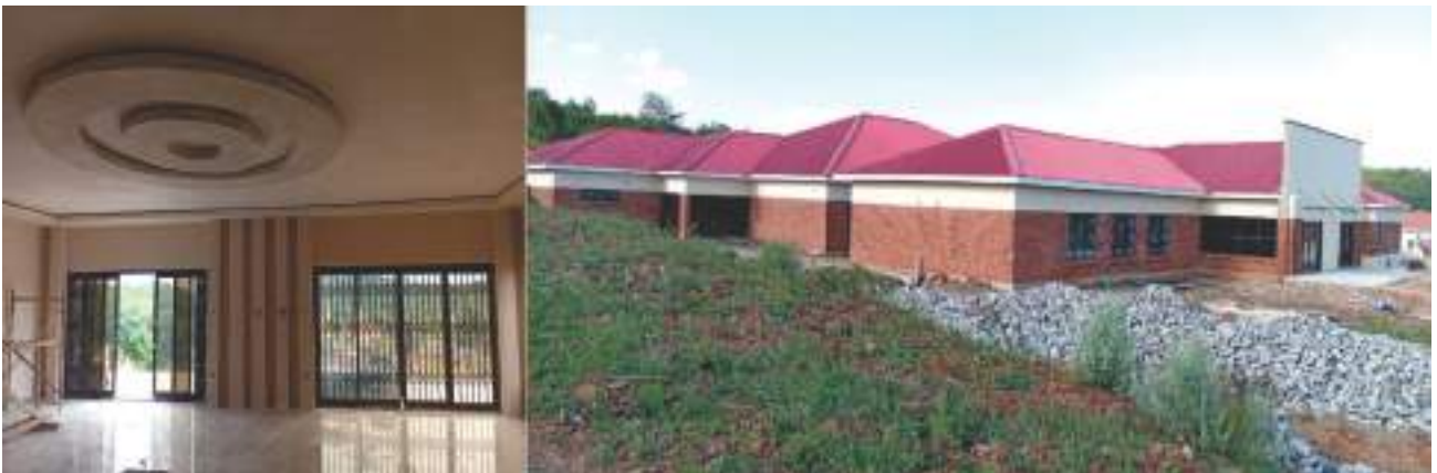
Gwanda State University-Agro and Technovation Complex
