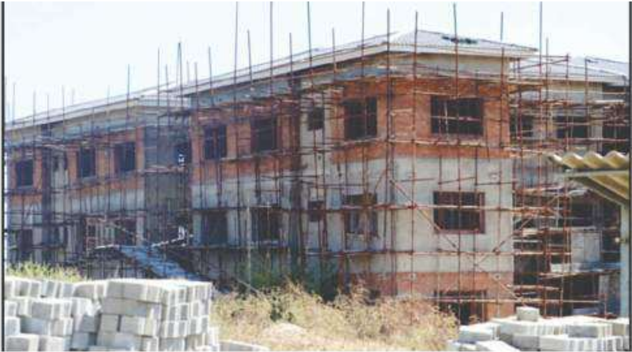
LSU 2 bedroomed Staff Flatlets (still under construction)
