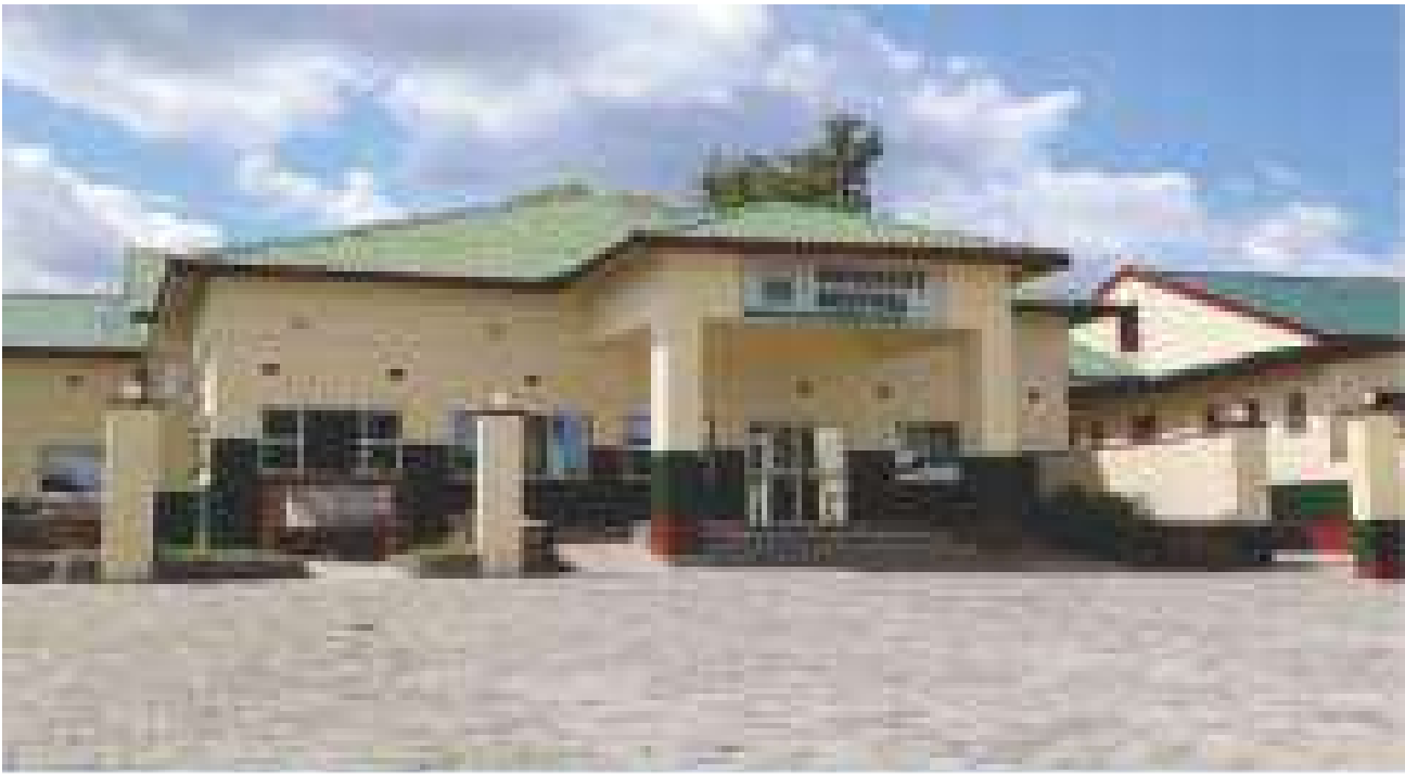
GZU Mashava Campus Hospital - Renovated old building with state of the art equipment for teaching.
